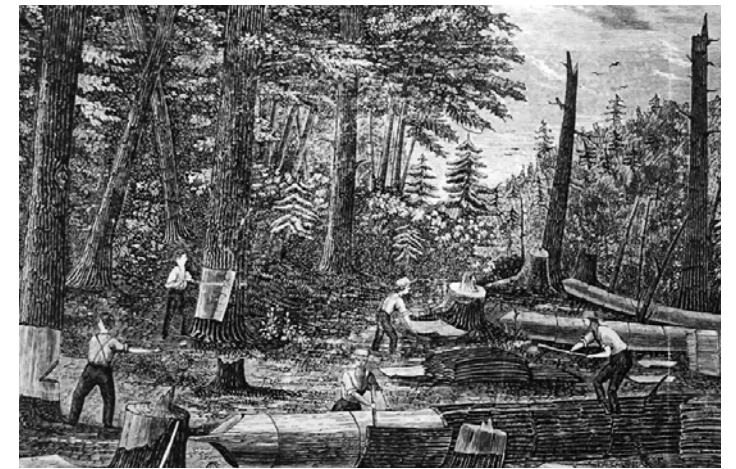
"Peeling, and piling hemlock bark, for Prattsville Tannery," ca. 1850
