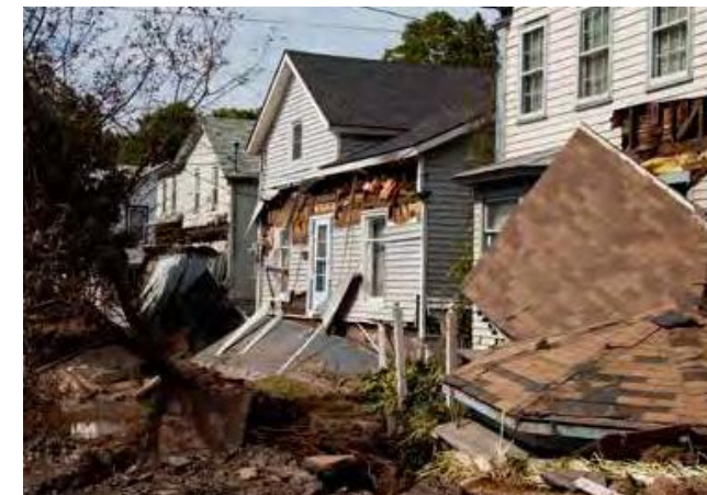
Houses destroyed after Hurricane Irene
