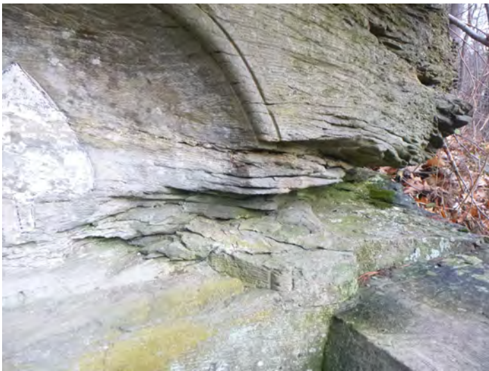
147-20 Stone_Spall Missing 2021-2
