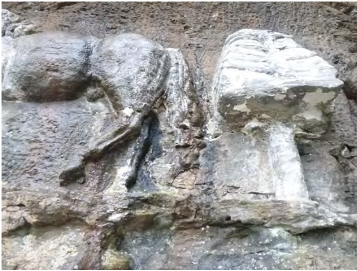
2-12 Stone_Spall Missing 2021-1
