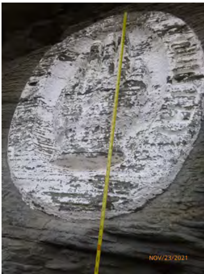
21-22 Stone_SurfLoss Eroded 2021-3
