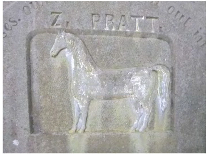
145-27 Stone_Coating Coating Failed 2021-2
