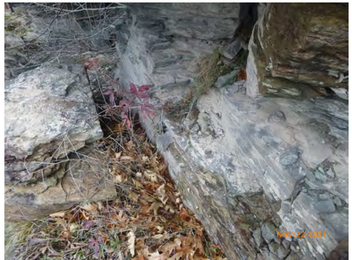
22-34 Stone_Note Photo-fissure above carving 2021-4
