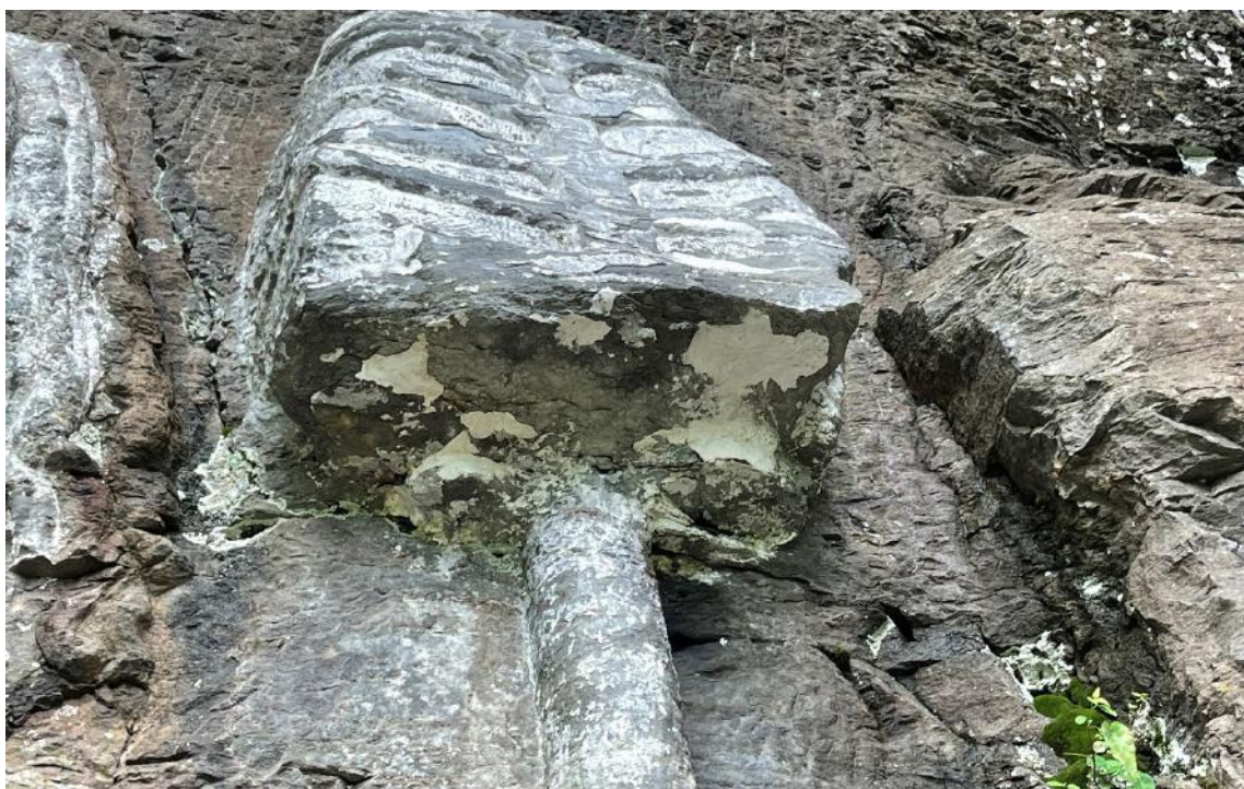
Figure 2: "Hemlock Tree" Sculpture, Coating Sample 2-3 Locations Coating samples 2-3 were obtained by ICR on 8/28/21 at the tree trunk and underside of the branches respectively.
