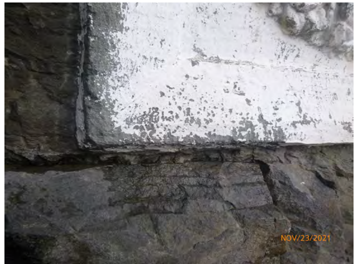
58-11 Stone_SurfLoss Eroded 2021-2
