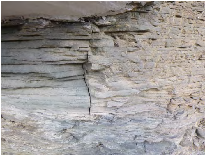
42-22 Stone_Crack Single unit 2021-1
