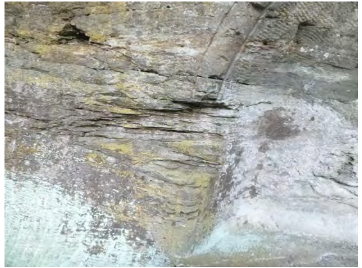
146-20 Stone_Spall Missing 2021-1
