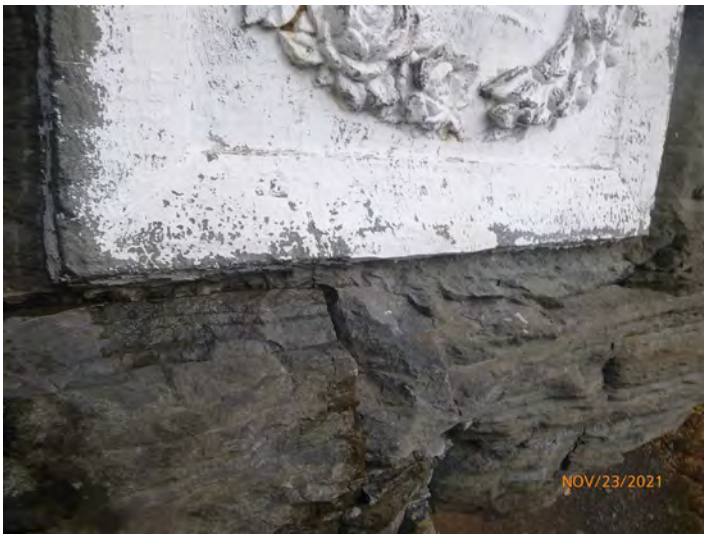
58-11 Stone_SurfLoss Eroded 2021-1
