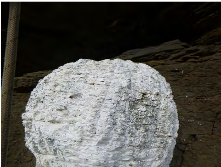
41-27 Stone_Coating Coating Failed 2021-1
