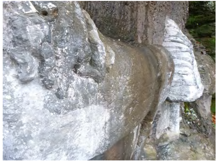
0-13 Stone_SurfLoss Eroded 2021-4
