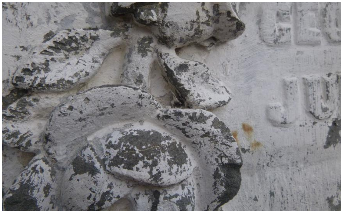
Figure 7: "Plaque to George and Julia Pratt," Coating Sample 8 Location Coating sample was obtained by VA on 11/22/21 from the left side of the sculpture.
