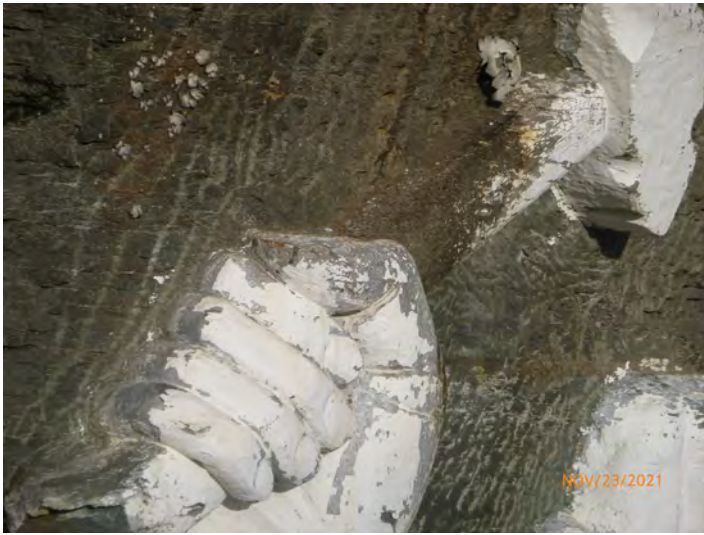
48-12 Stone_Spall Missing 2021-1
