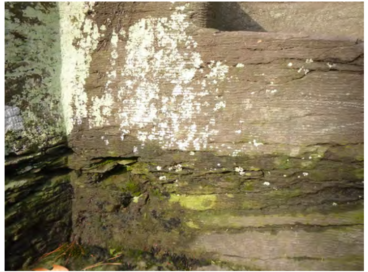
168-20 Stone_SurfLoss Eroded 2021-7
