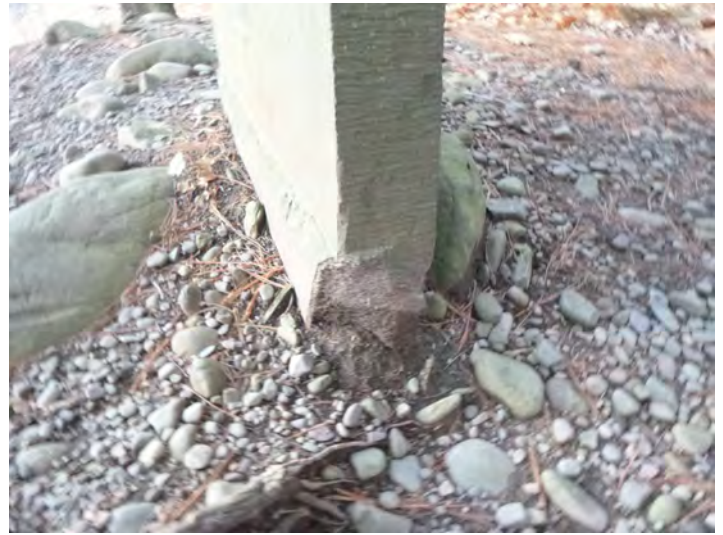
146-24 Stone_Spall Missing 2021-2
