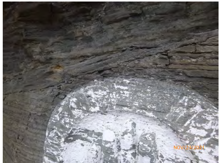
23-25 Stone_SurfLoss Delaminated 2021-1
