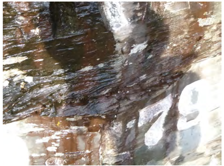
39-13 Stone_Crack Single unit 2021-1
