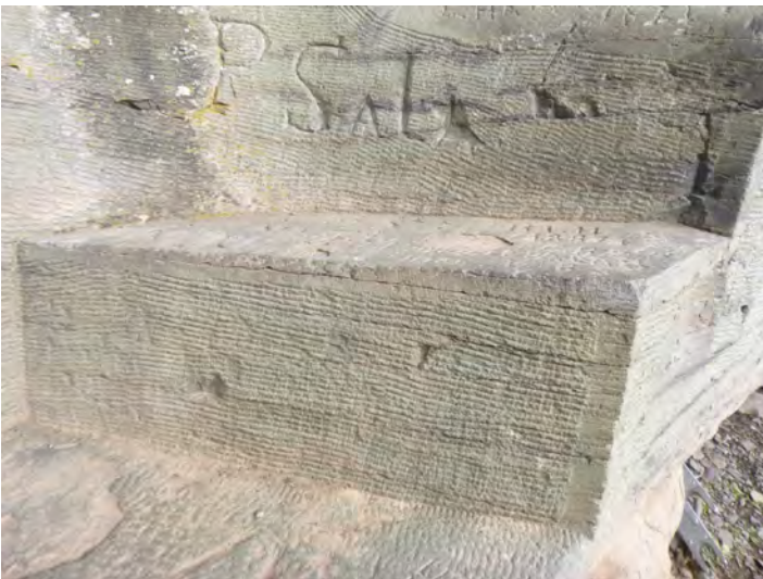
139-14 Stone_SurfLoss Delaminated 2021-1
