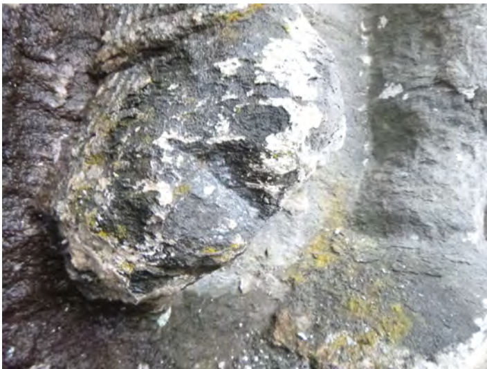
2-11 Stone_Spall Missing 2021-2
