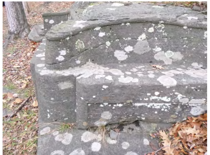
162-25 Stone_Spall Missing 2021-2
