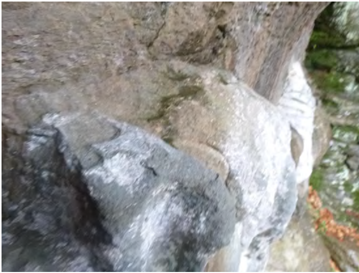
0-13 Stone_SurfLoss Eroded 2021-3
