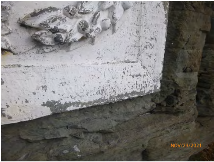
58-11 Stone_SurfLoss Eroded 2021-3
