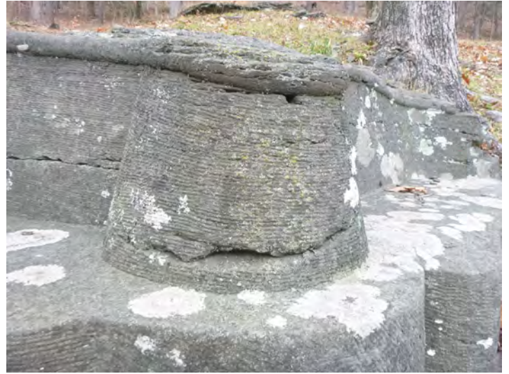
161-26 Stone_Crack System units 2021-3
