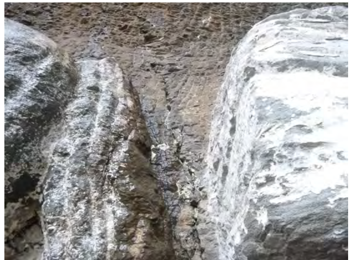
3-13 Stone_Crack System units 2021-1
