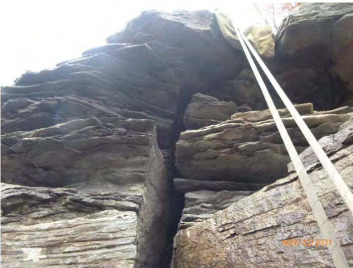
22-34 Stone_Note Photo-fissure above carving 2021-1
