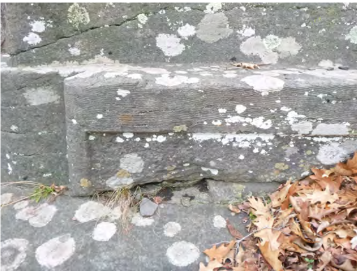
162-25 Stone_Spall Missing 2021-1
