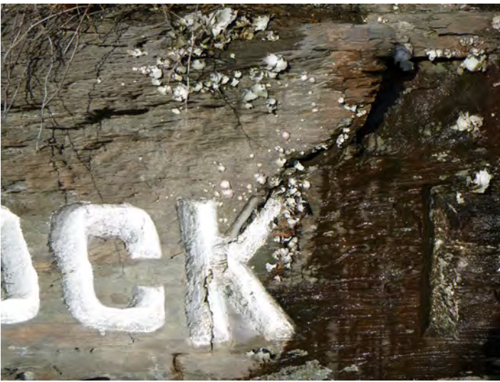
37-17 Stone_Crack Single unit 2021-1
