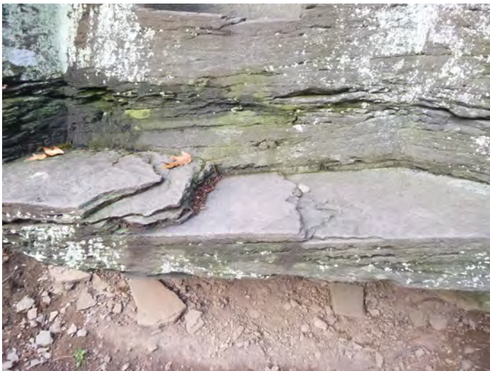
168-20 Stone_SurfLoss Eroded 2021-2
