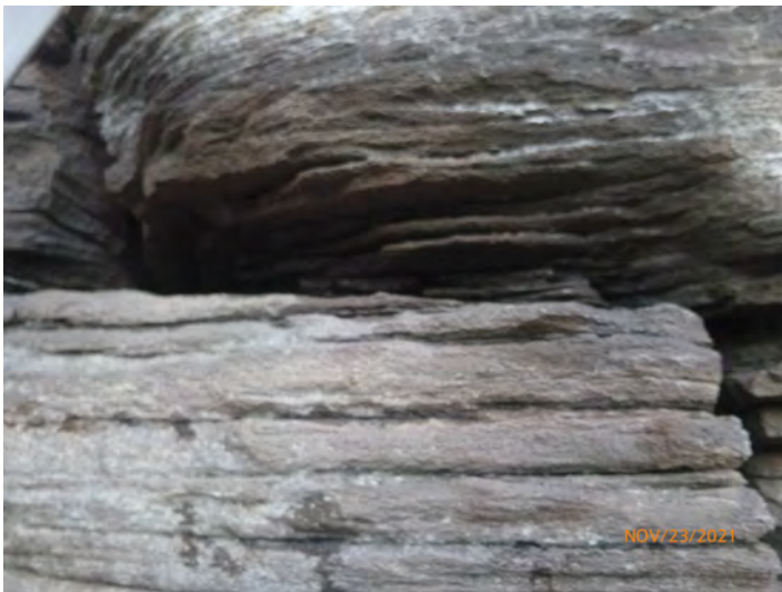
54-15 Stone_Crack Single unit 2021-2
