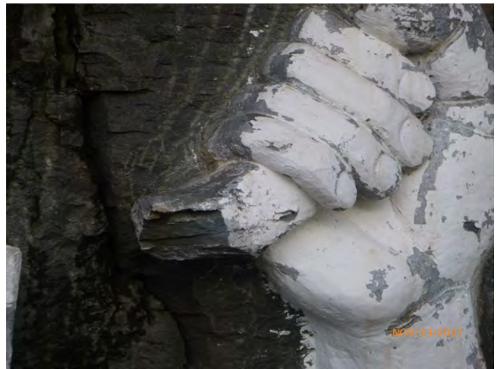
48-11 Stone_Spall Missing 2021-1
