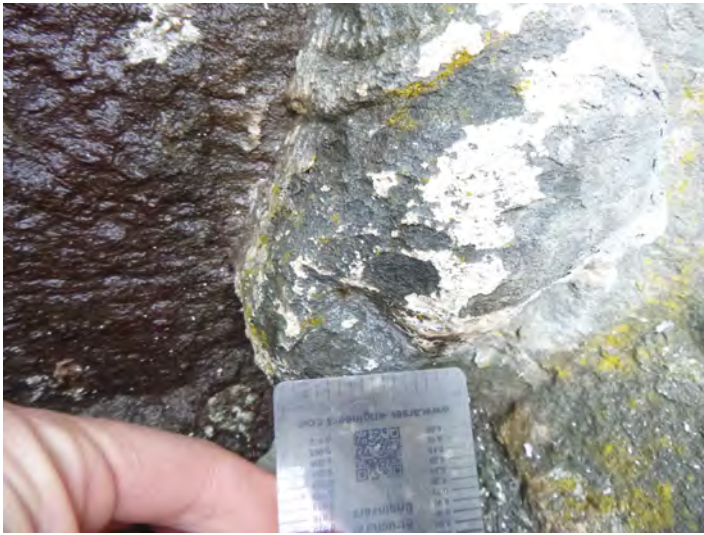
2-11 Stone_Spall Missing 2021-4
