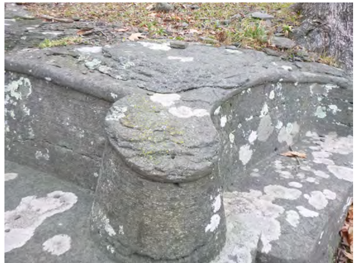
161-26 Stone_SurfLoss Eroded 2021-1
