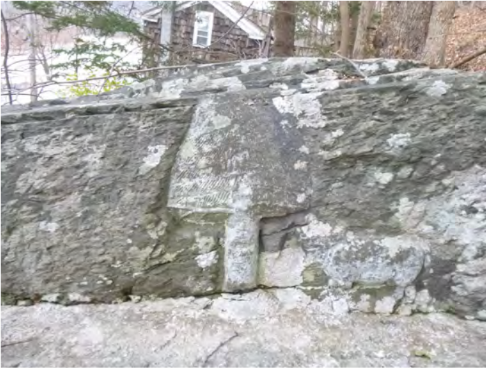
169-26 Stone_Spall Missing 2021-1
