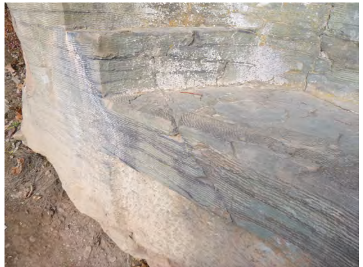
137-14 Stone_Crack System units 2021-1
