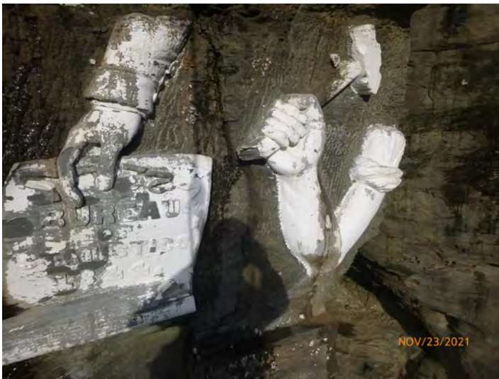
50-8 Stone_Crack Single unit 2021-2
