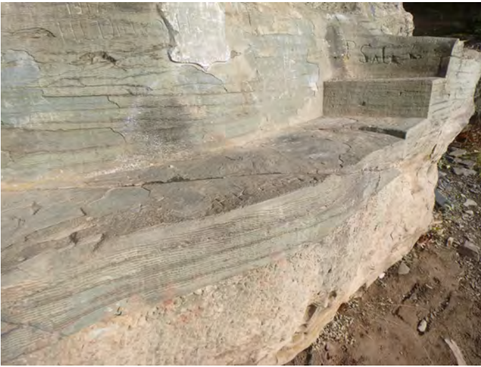
139-14 Stone_Crack System units 2021-2
