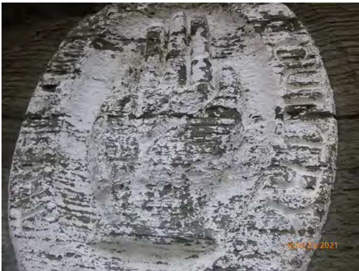
21-22 Stone_SurfLoss Eroded 2021-1
