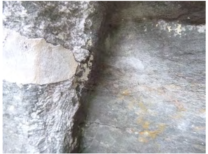
1-12 Stone_Repair Patch Sound 2021-3
