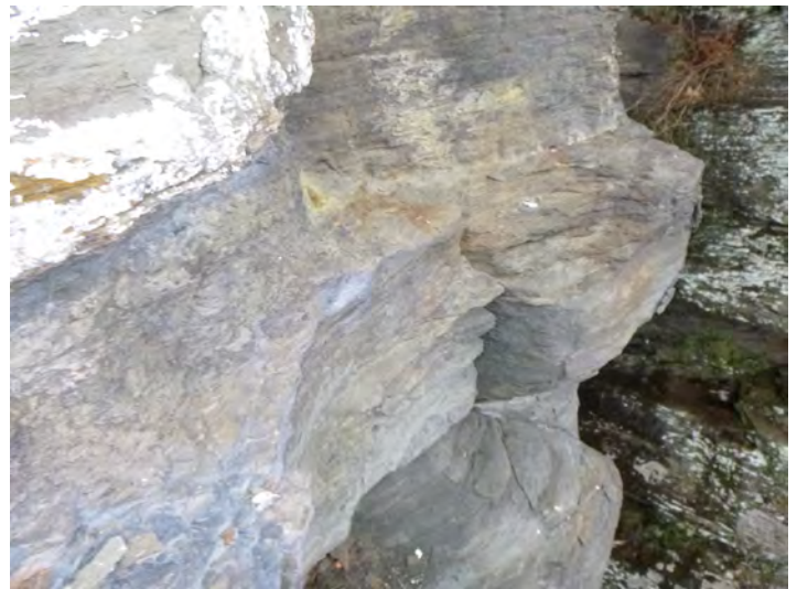
17-17 Stone_Crack Single unit 2021-1
