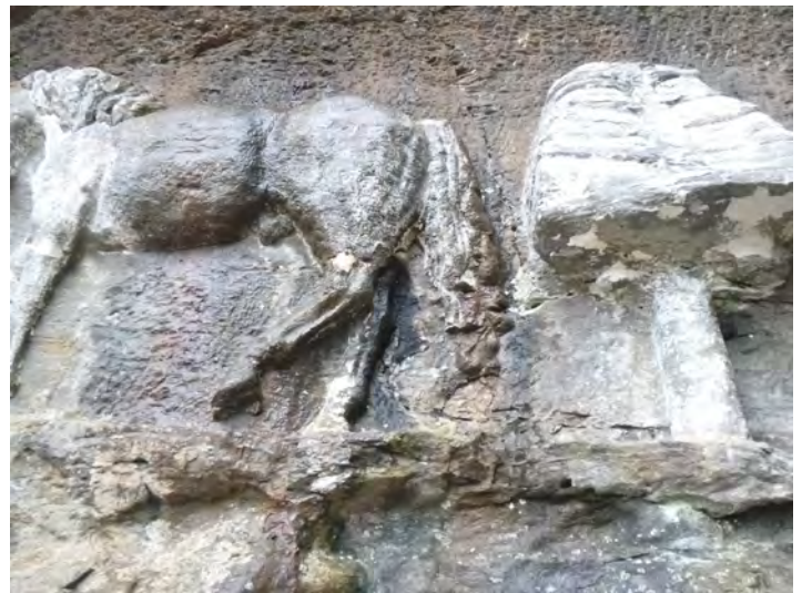
5-11 Stone_Note Photo-water seepage 2021-1
