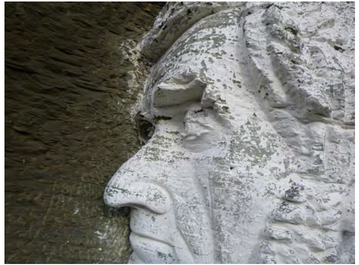
41-27 Stone_Coating Coating Failed 2021-4
