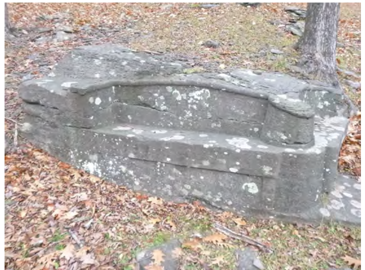
161-26 Stone_Crack System units 2021-1
