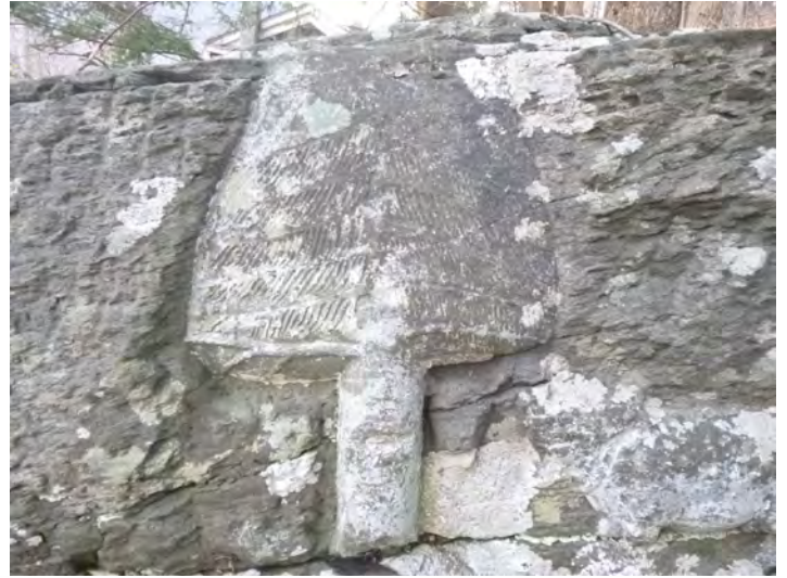
169-26 Stone_SurfLoss Eroded 2021-1
