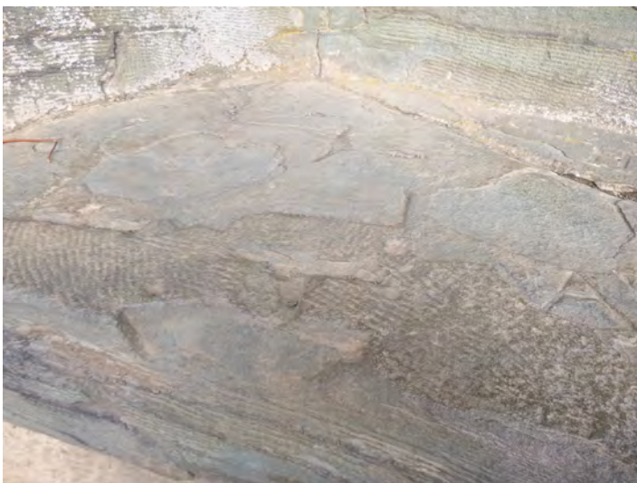
137-14 Stone_SurfLoss Delaminated 2021-1
