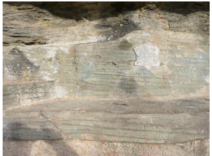
139-14 Stone_Crack System units 2021-1
