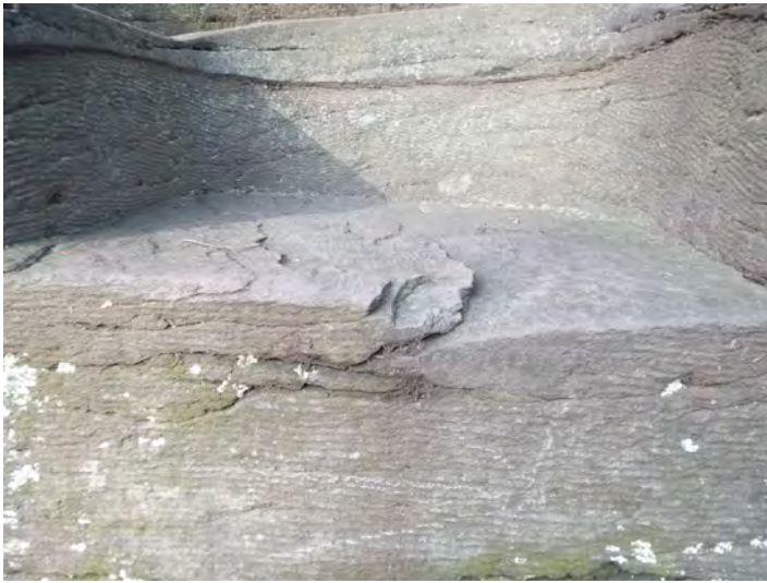
168-20 Stone_SurfLoss Eroded 2021-6
