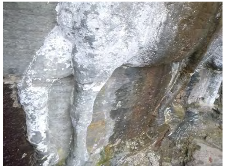
1-12 Stone_Repair Patch Sound 2021-1
