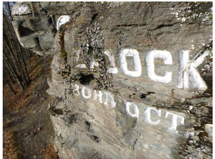
36-14 Stone_Coating Coating Failed 2021-1
