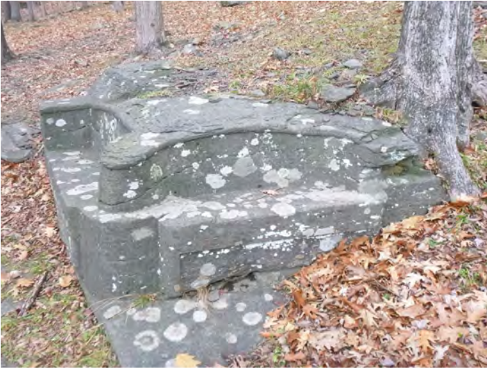
161-26 Stone_Crack System units 2021-2
