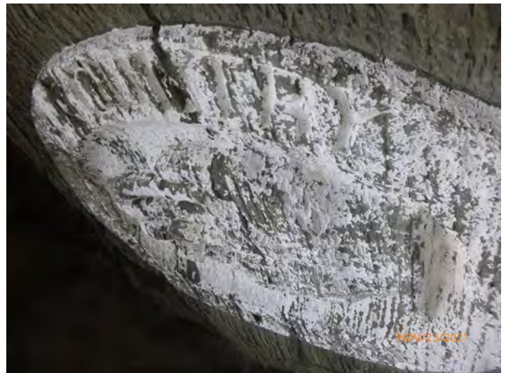
21-22 Stone_SurfLoss Eroded 2021-2
