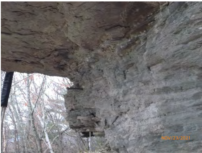
19-27 Stone_Embedment Ferrous Embedment 2021-1
