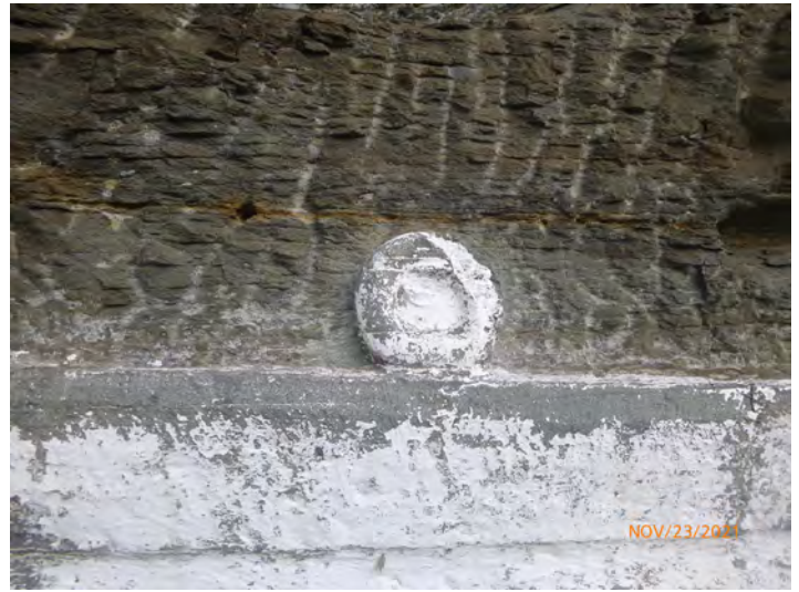
58-16 Stone_Spall Missing 2021-1
