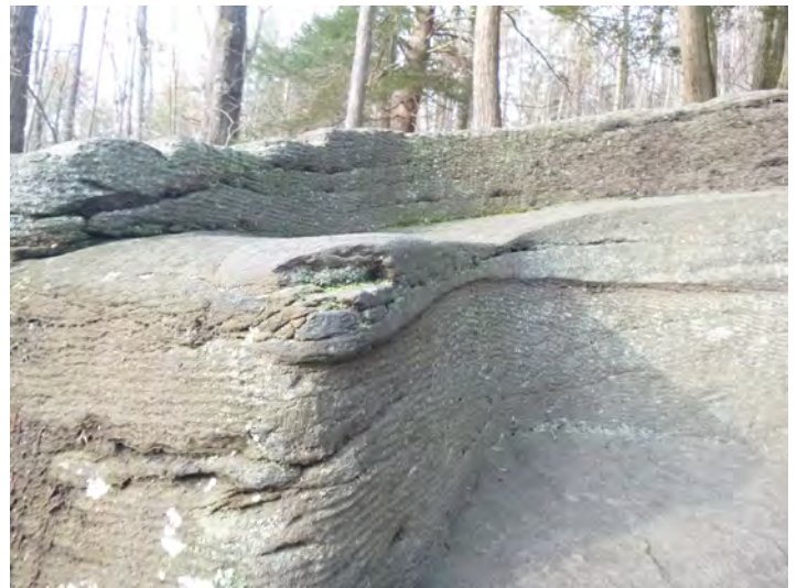
168-20 Stone_SurfLoss Eroded 2021-5
