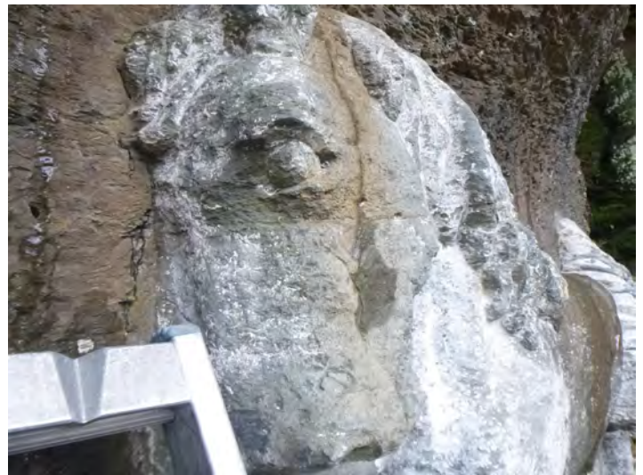
0-12 Stone_Coating Coating Failed 2021-6
