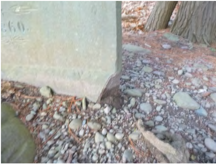
146-24 Stone_Spall Missing 2021-1
