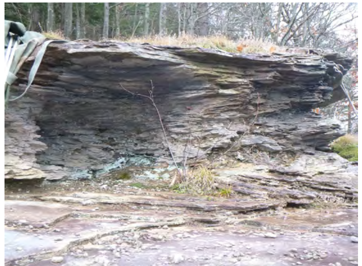
13-39 Stone_Note Photo- undermined 2021-2
