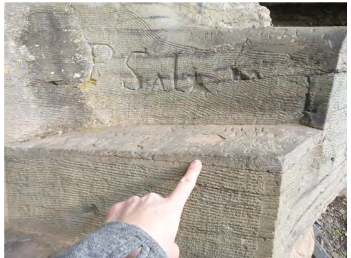
139-14 Stone_SurfLoss Delaminated 2021-2
