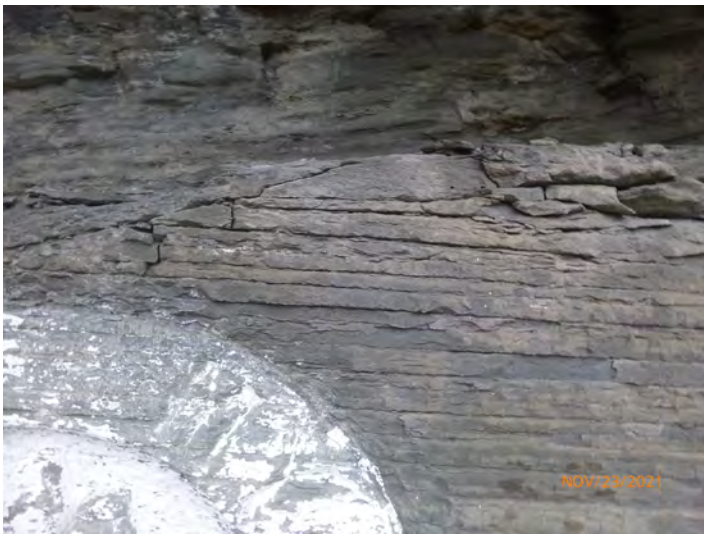
23-25 Stone_SurfLoss Delaminated 2021-2
