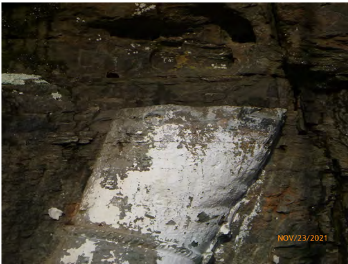
47-13 Stone_Spall Missing 2021-1
