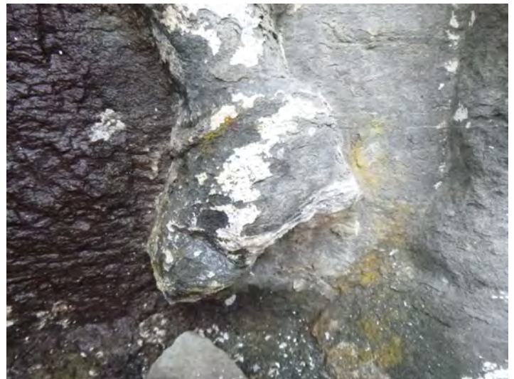
2-11 Stone_Spall Missing 2021-1
