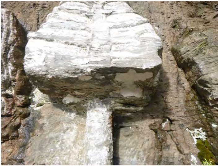
4-12 Stone_Spall Missing 2021-1
