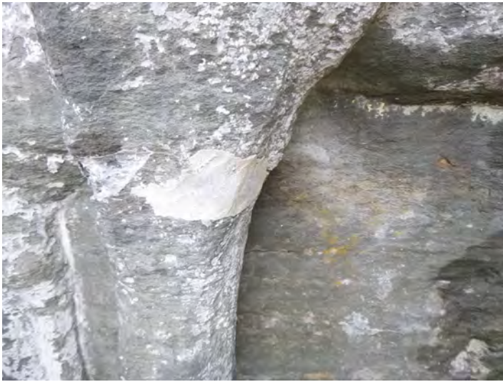
1-12 Stone_Repair Patch Sound 2021-2
