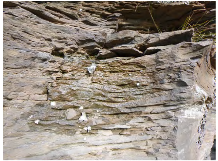
43-27 Stone_Note Photo- Water seepage 2021-1
